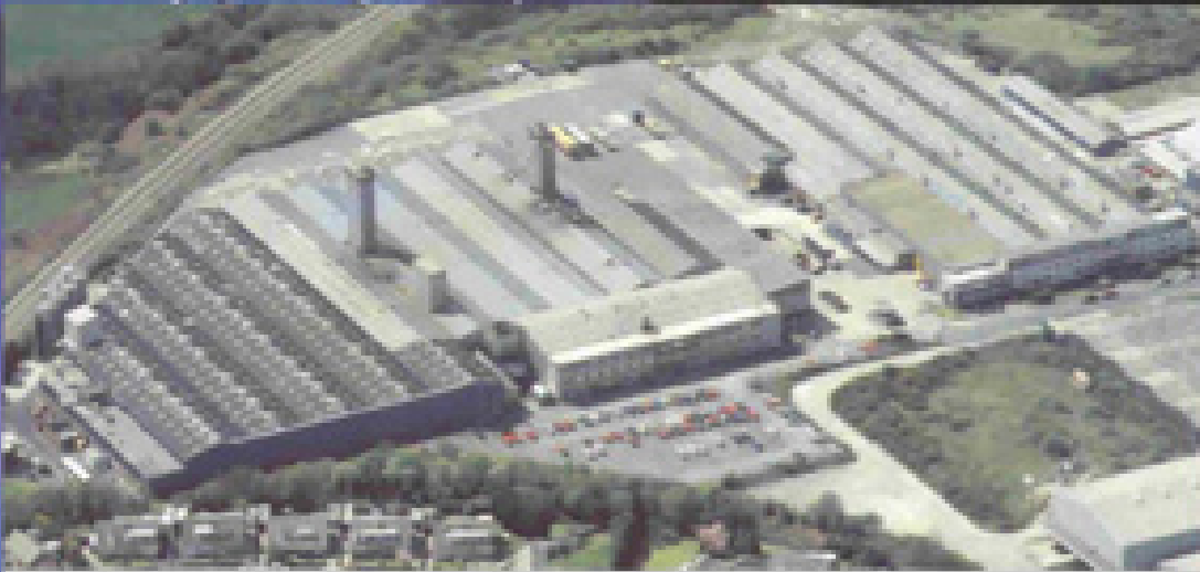
One of the many manufacturing facilities operated by Signode throughout Europe and worldwide.
